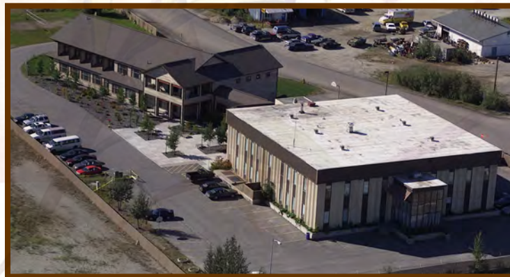
Aerial view of the Ralph Perdue Center
